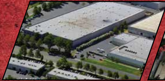
Manufacturing Facility - West Sacramento, California
